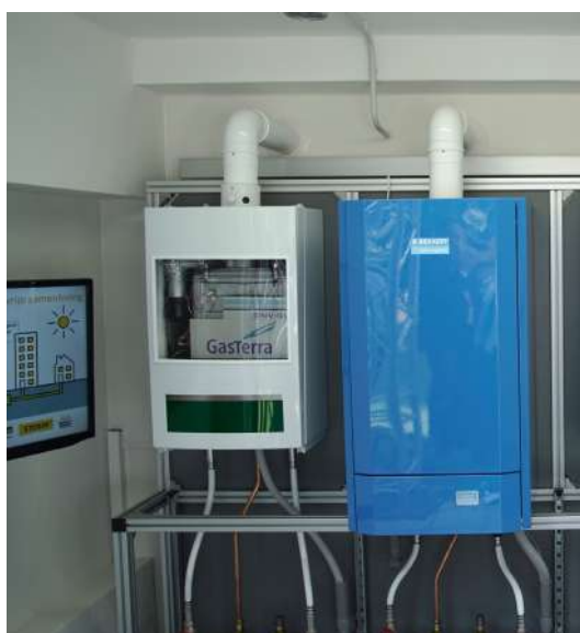
Figure 4 - Left: DNV GL/Gasterra (boiler 1) and Bekaert (boiler 2) condensing boilers in Rozenburg demonstration Right: NO x emission measured in hydrogen boiler 1 & 2 at different thermal loads
